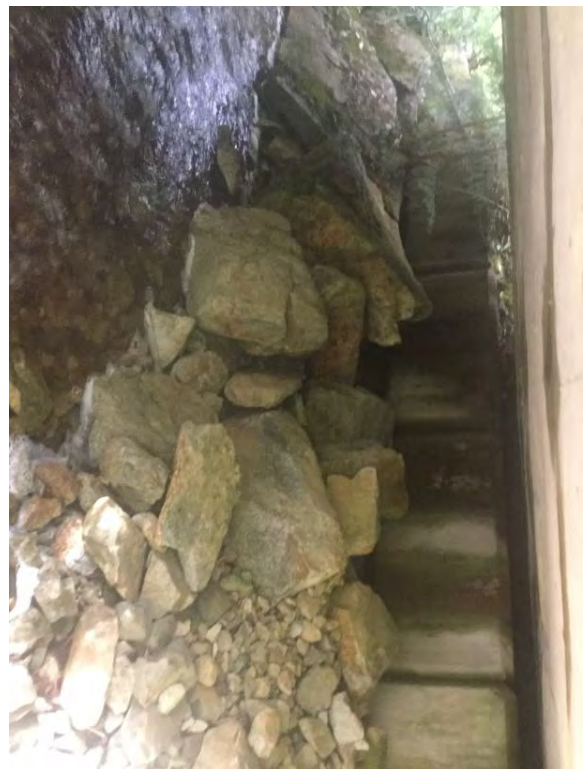
Right Bank Abutment when facing downstream
